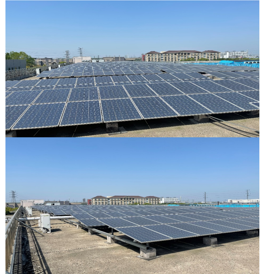
300w photovoltaic power generation facilities in Wujiang Plant
